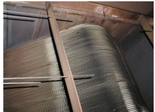
(b) After Removal of Soot by Air Bypass
