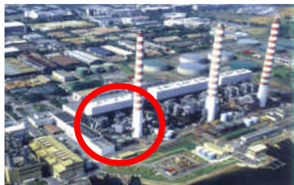
Fig 15: Aerial view of Senoko Power Plant (space for Repowering phase 1 &amp; 2 is marked red)
