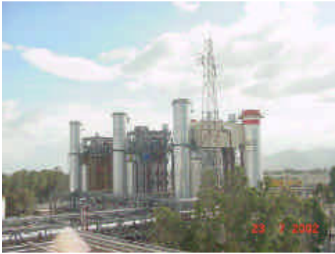
Fig 14: Valle de Mexico power plant
