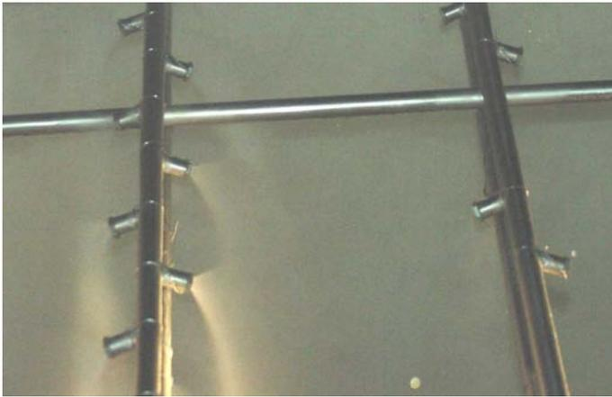
Figure 2 High Fogging rack spraying at reduced mass flow into the intake manifold of the GT8C2 during gas turbine operation (at plane C in Figure 1).
