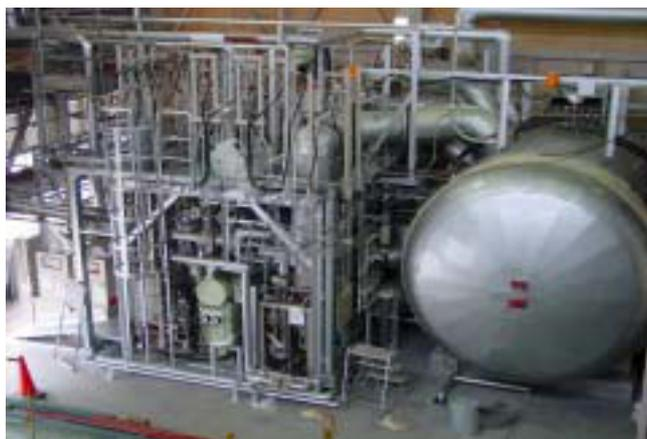
Figure 6 Installation of pressurized compact system at Kawagoe site
