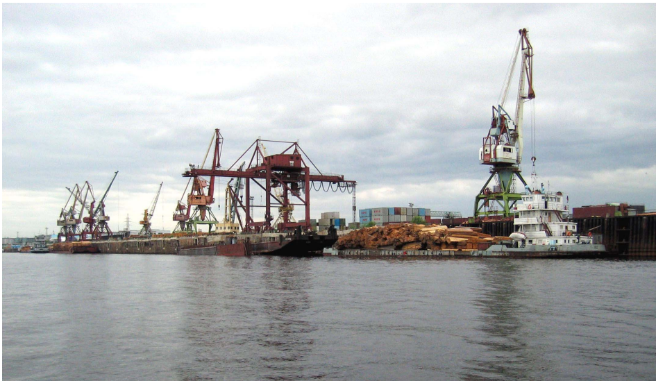
Figure 4 Cargo Handling Facilities on the Lena River
