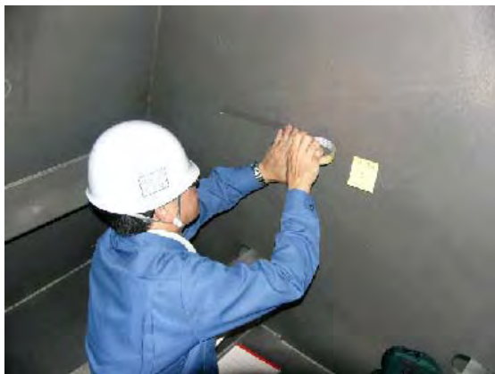
Photo.1 Dust measurement on the wall surface
