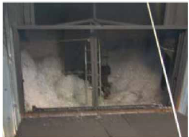
98 seconds after Foam discharge. The fire extinguished completely.
