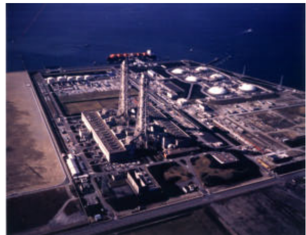
Fig. 1 TEPCO Futtsu Thermal Power Station
